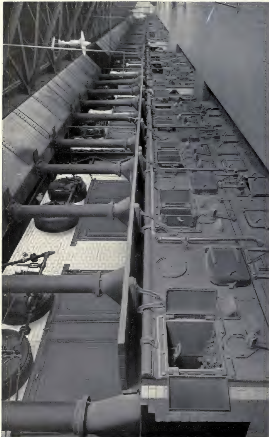
CAMBRIA STEEL CO., JOHNSTOWN, PA. 4880 HORSE POWER OF BABCOCK & WILCOX BOILERS, EQUIPPED WITH BABCOCK & WILCOX SUPERHEATERS. THIS COMPANY HAS BABCOCK & WILCOX SUPERHEATERS INSTALLED IN 26,700 HORSE POWER OF BABCOCK & WILCOX BOILERS
